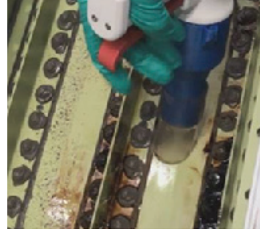
Image 3: After the sanitization and comprehensive removal of biofilm build-up.
